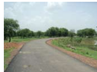
Bituminous Road at Murethi
